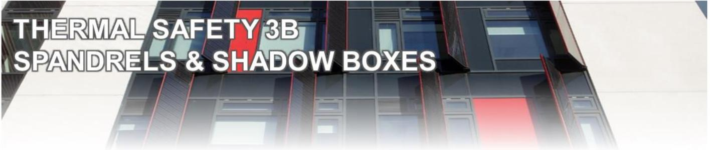
Spandrels and shadow boxes are typically used to conceal regions of the building containing utilities (pipes/cables) or structural elements, whilst still maintaining the appearance of a full glass façade. Spandrel units will typically have an opaque pane, and insulation in contact with the rear of the glazing unit, either adhered to the glass or secured in metal trays.
